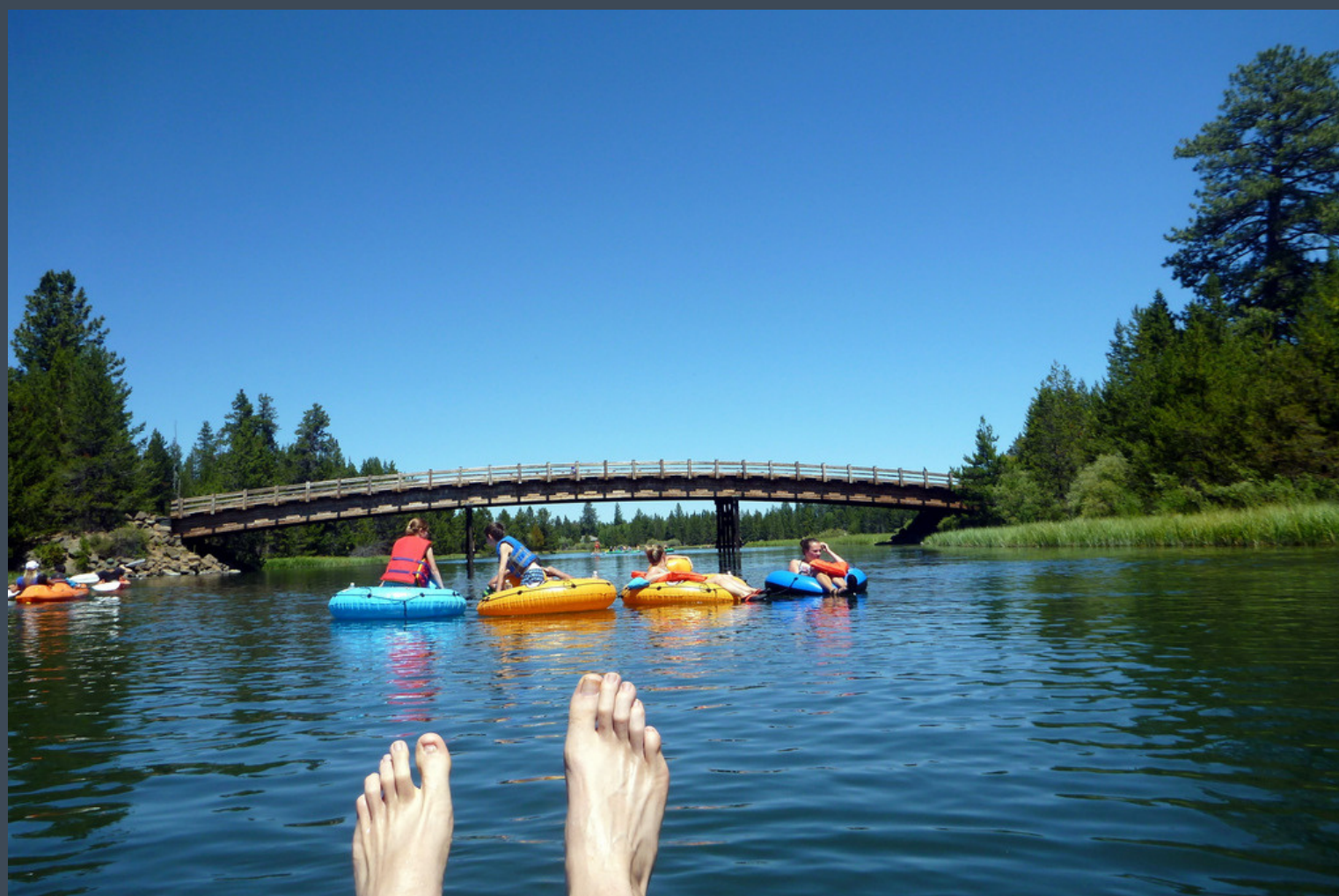
Cardinal Landing Foot Bridge
